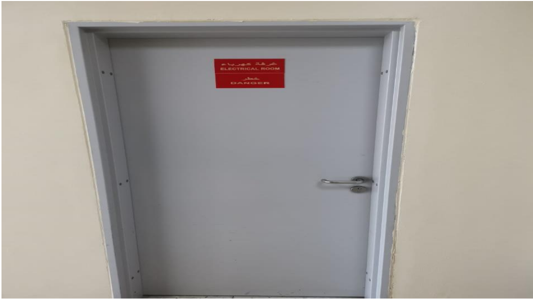
Photo 4: Shows USTF electrical rooms and electric boxes have a displayed hazard warning sign
