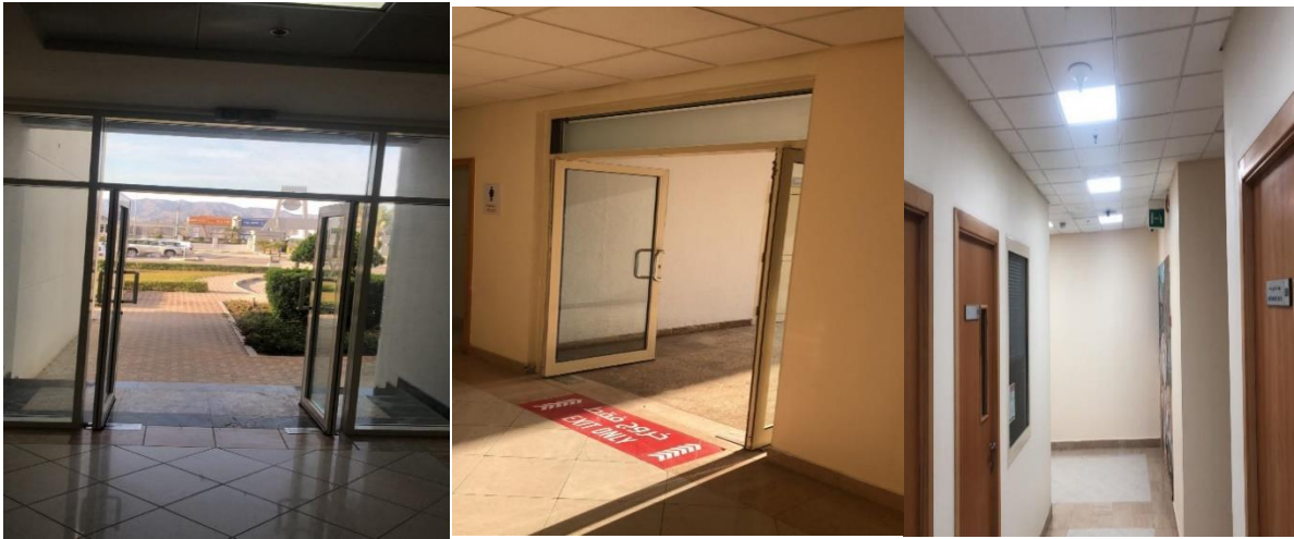
Photo 11: Shows access to-and the integrity of all USTF external and internal areas are maintained
