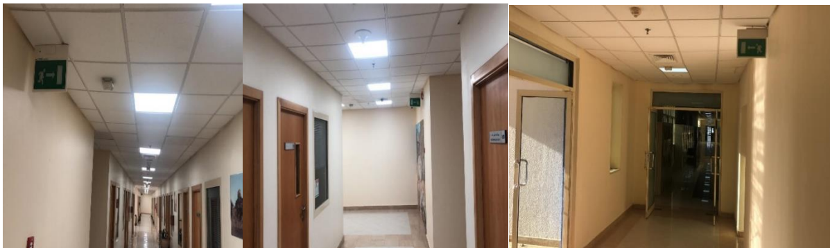
Photo 13: Shows USTF maintain an easily enough accessed emergency exits fitted with illuminated signs at exits/emergency doors
