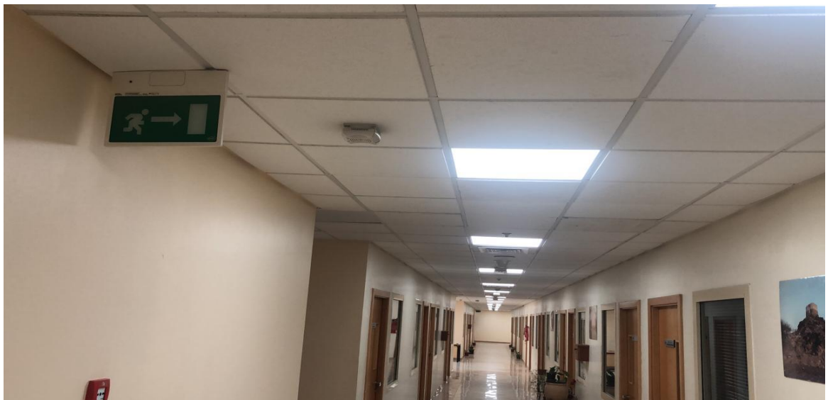
Photo 2: Shows USTF has illuminated 'Emergency Exit' signs
