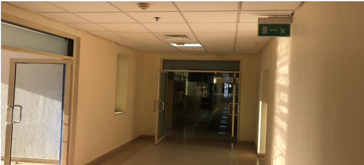
Photo 1: Shows USTF has illuminated 'Emergency Exit' signs
