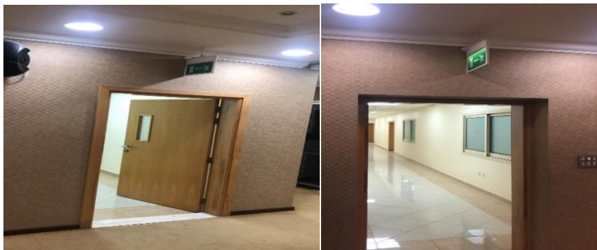
Photo 8: Shows USTF auditorium has additional emergency exit behind the stage
