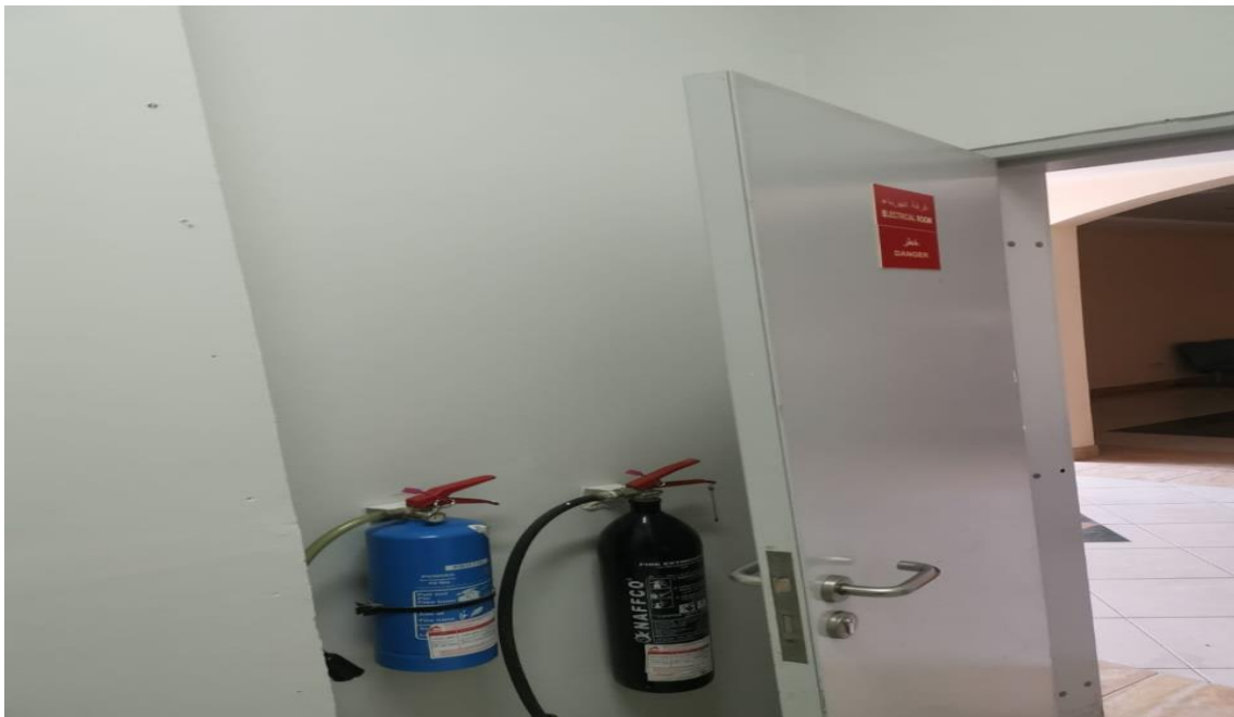
Photo 3: Shows USTF electrical rooms maintained with operational fire extinguishers
